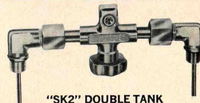
"SK2" DOUBLE TANK MANIFOLD
